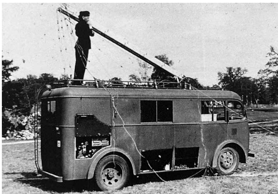
Markradiostation Tmr VIII, mast under resning.
